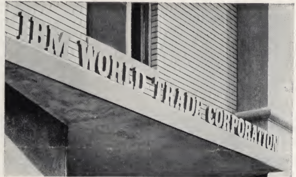
L-8: Special logotype fabricated of sheet stainless steel and mounted on a flat bar for attachment to canopy.
